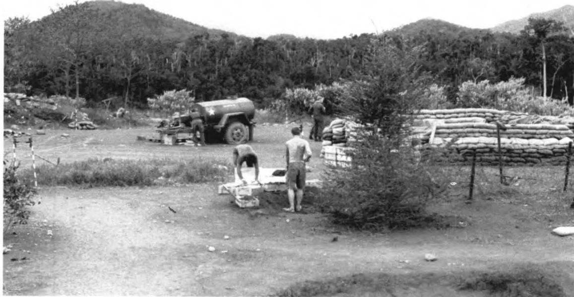
Kodak Ektachrome slide, Roll 1, Number 7. [printed as digital black and white photograph]. Two soldiers filling ammo boxes with dirt for bunkers. Water supply tank ["water buffalo"], to left of center.
