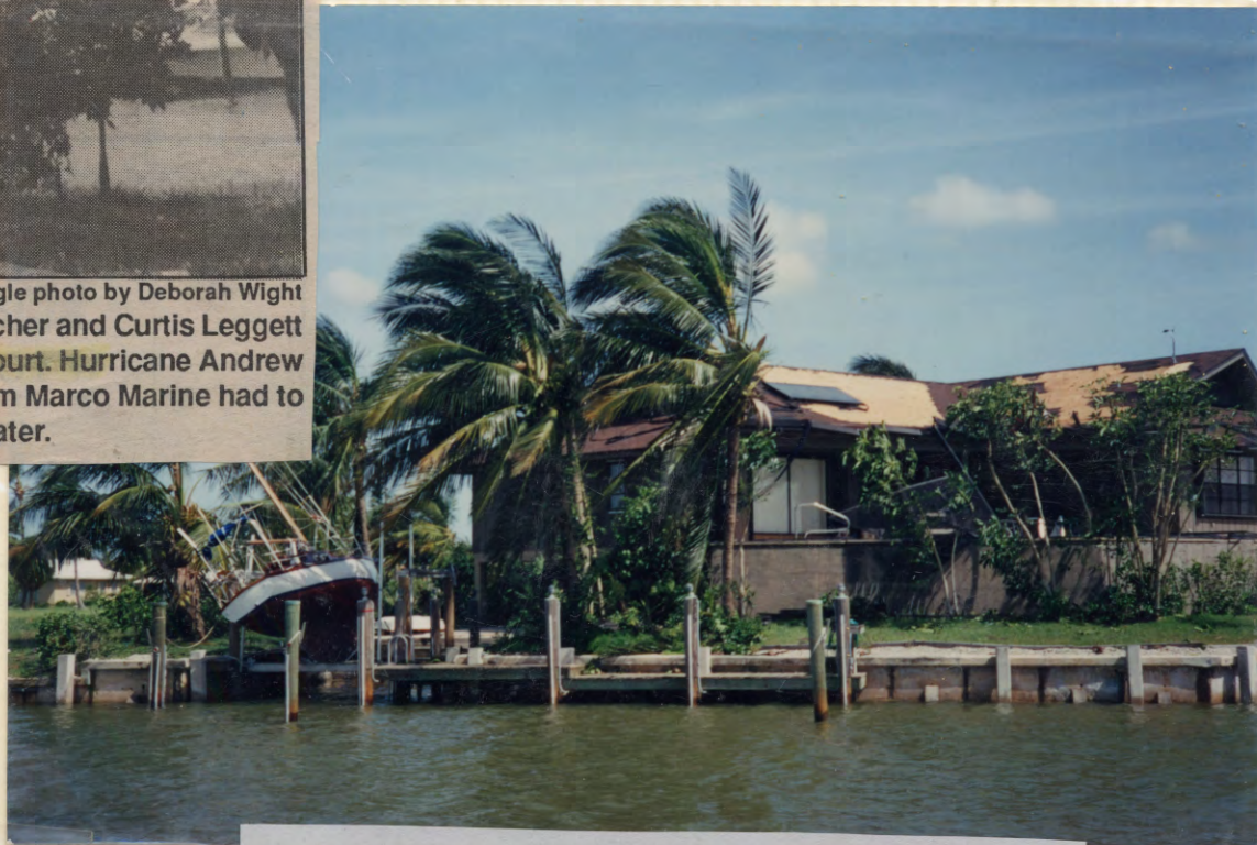
Jesse's house after the hurricane.
