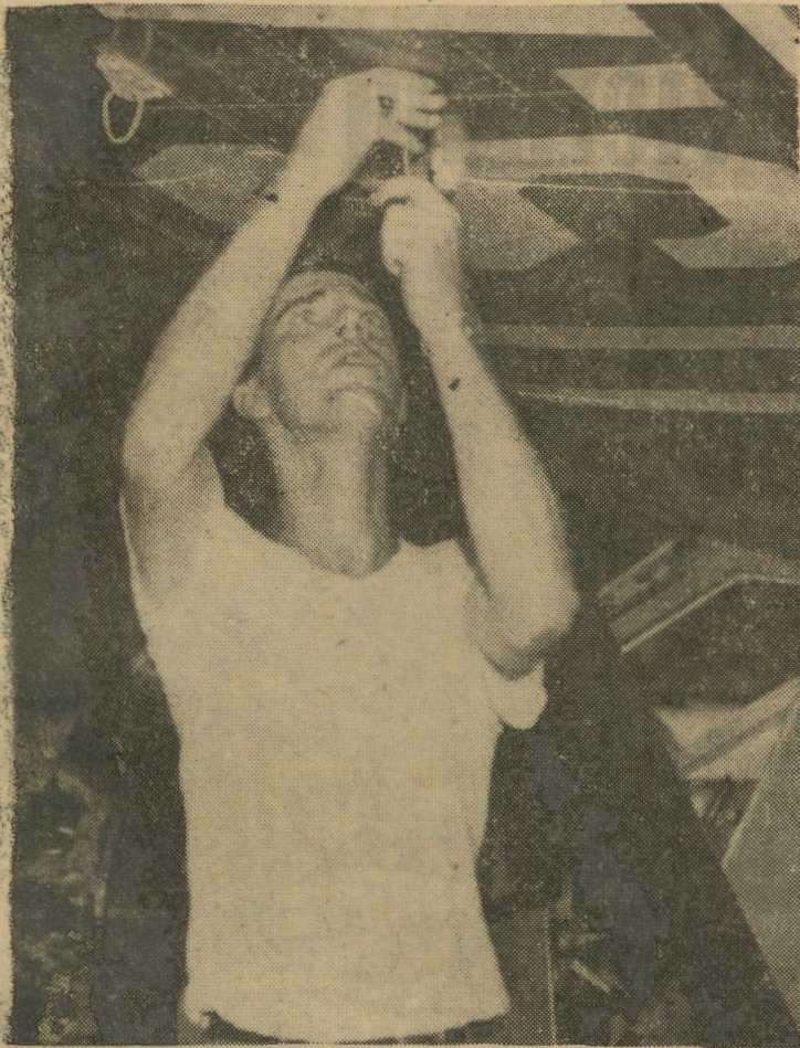
READY TO ROLL — Sp4 John L. Iuhan, a crew chief, replaces plates on the wing of a U-6 after completing periodic inspection, which lasts about three days.
