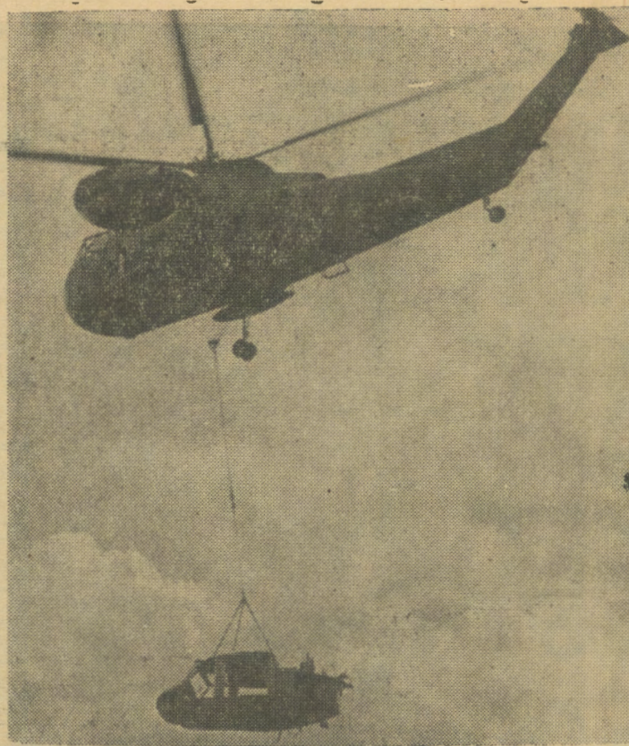
ON THE WAY — A twin-engined Mohave H-37 helicopter easily lifts the hulk of a "huey" from the site where it crashed and returns it to base where parts of it may be salvaged. Members of the 56th Transportation Company fly the huge choppers into zones where other copters have crashed to salvage the craft if possible but mainly to deprive the VC of parts and equipment on the crashed bird.
