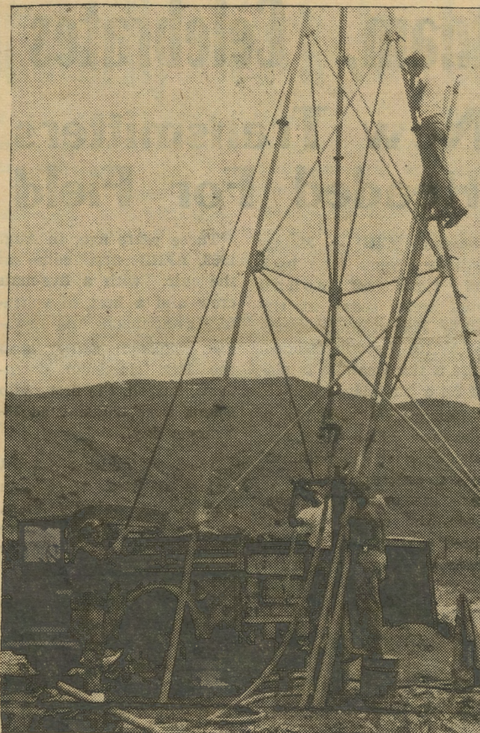
HOMEMADE — Mobile Construction Battalion 3's well drilling team works on their homemade drilling rig near Da Nang. When the team's $35,000 drilling rig broke down and they couldn't get parts for it, they built this rig themselves. It utilizes a jet stream of water that erodes away the dirt beneath the pipe stem allowing it to sink into the ground.
