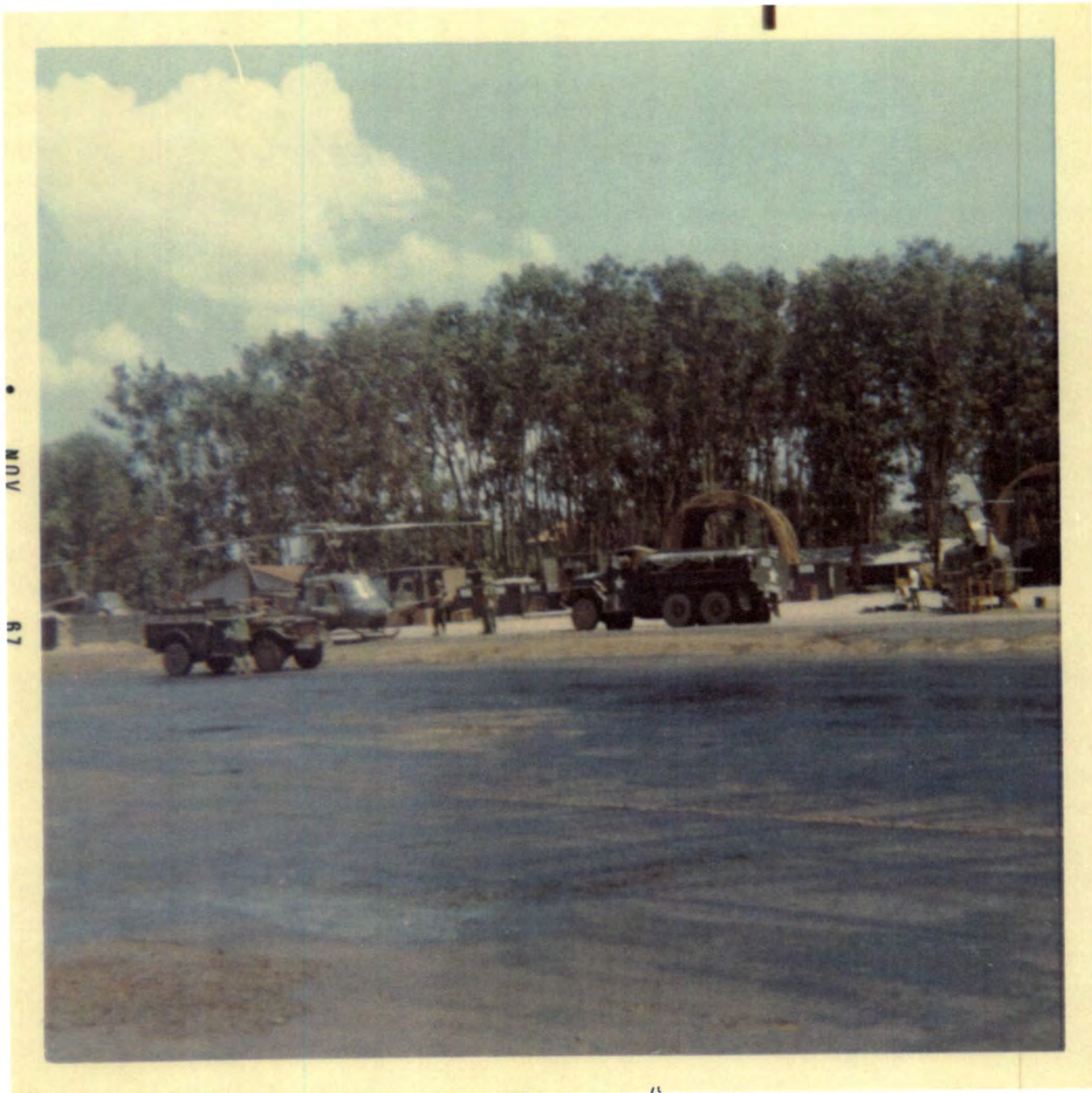
6031d MAINTENANCE RAMP @ THE "WEB"
