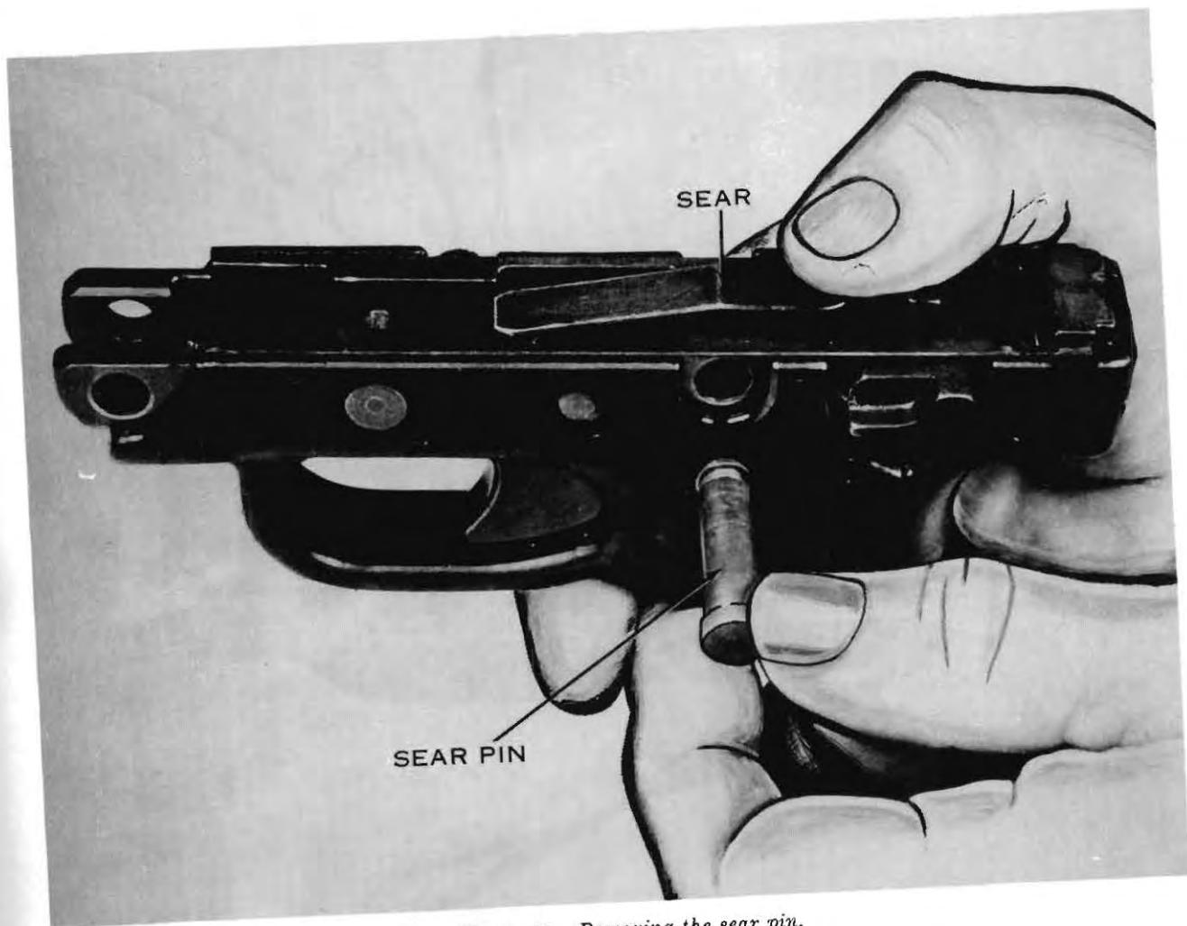
Figure 20. Removing the sear pin.
