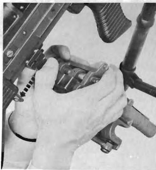
Figure 38. Removing the traversing and elevating mechanism.
