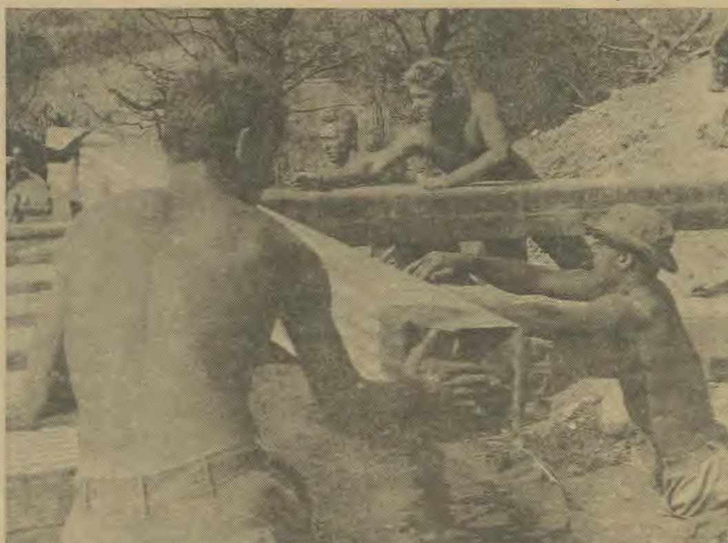
Three engineers push a piece of road surface material onto a pontoon bridge.
