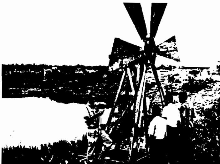
PETER HUNTING REPAIRS LOCALLY - MADE IRRIGATION WINDMILL.
