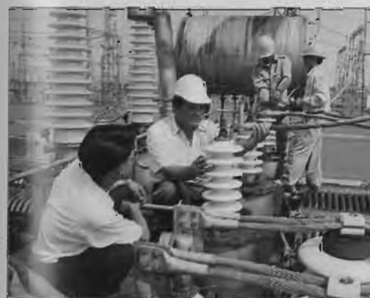
Repair of MBA T2, 220 KV station at Vinh
