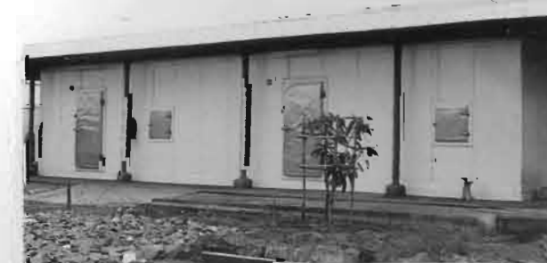
KHO LẠNH COLD STORAGE
