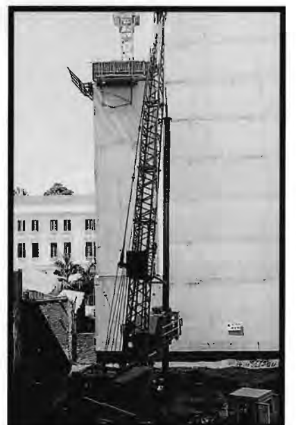
Bored Piling Work, Landmark Project 24 Trang Tien, Hanoi
