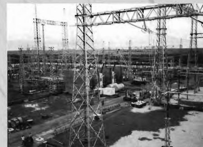
Lắp trạm 500/200KV - 2x450MVA Phú Lâm. Installation of Phú Lâm 500/200KV - 2x450MVA power substation.
