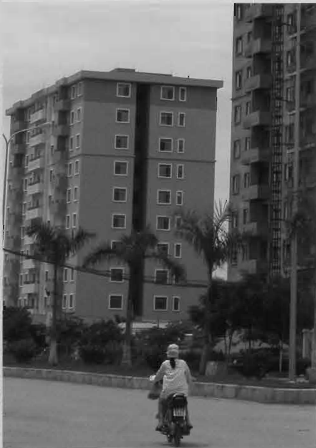
Part of the Van Quan-Yen Phuc New Urban Area in construction
