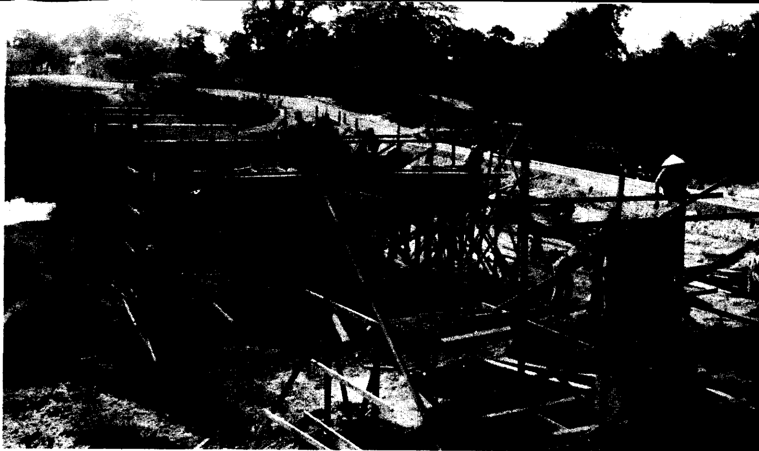
Workmen push ahead on bridge construction as part of National Route 21 project near Banmethuot
