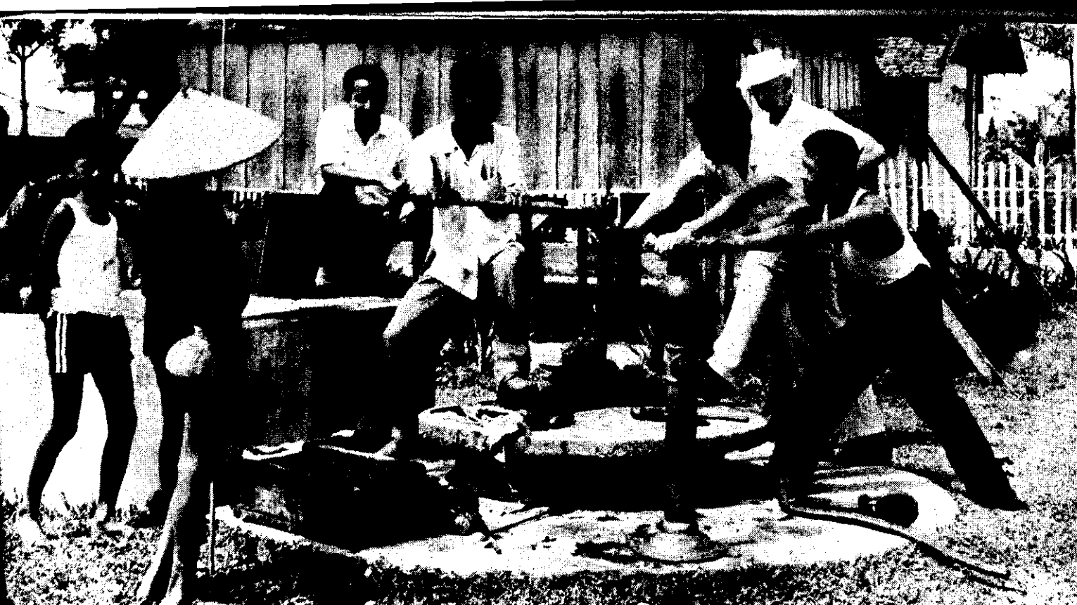
Once wells are drilled, local authorities are taught importance of pump repair and maintenance
