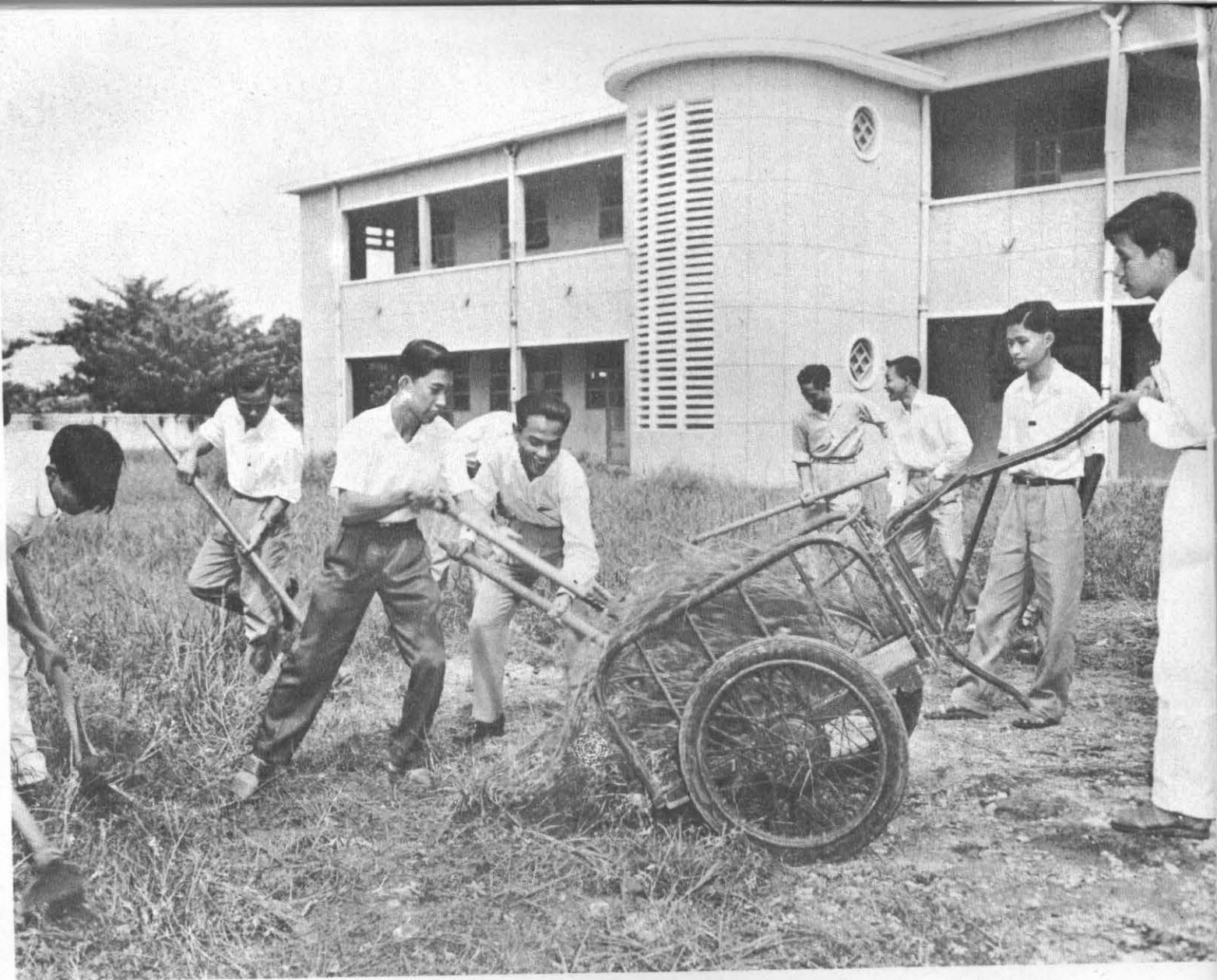
Students pitch in to clean up Normal School grounds. School was built with American Aid funds
