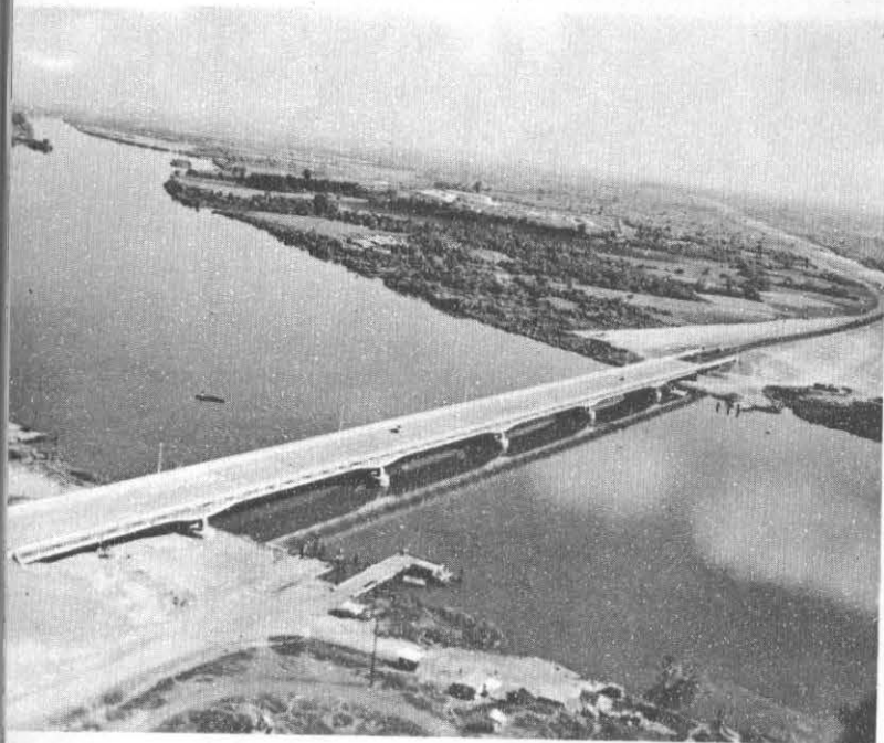
The Dong-Nai River Bridge, second longest in Vietnam, on the Saigon-Bien-Hoa Highway.
