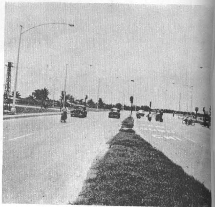
The new Saigon-Bien-Hoa Highway at the Hung-Vuong intersection.
