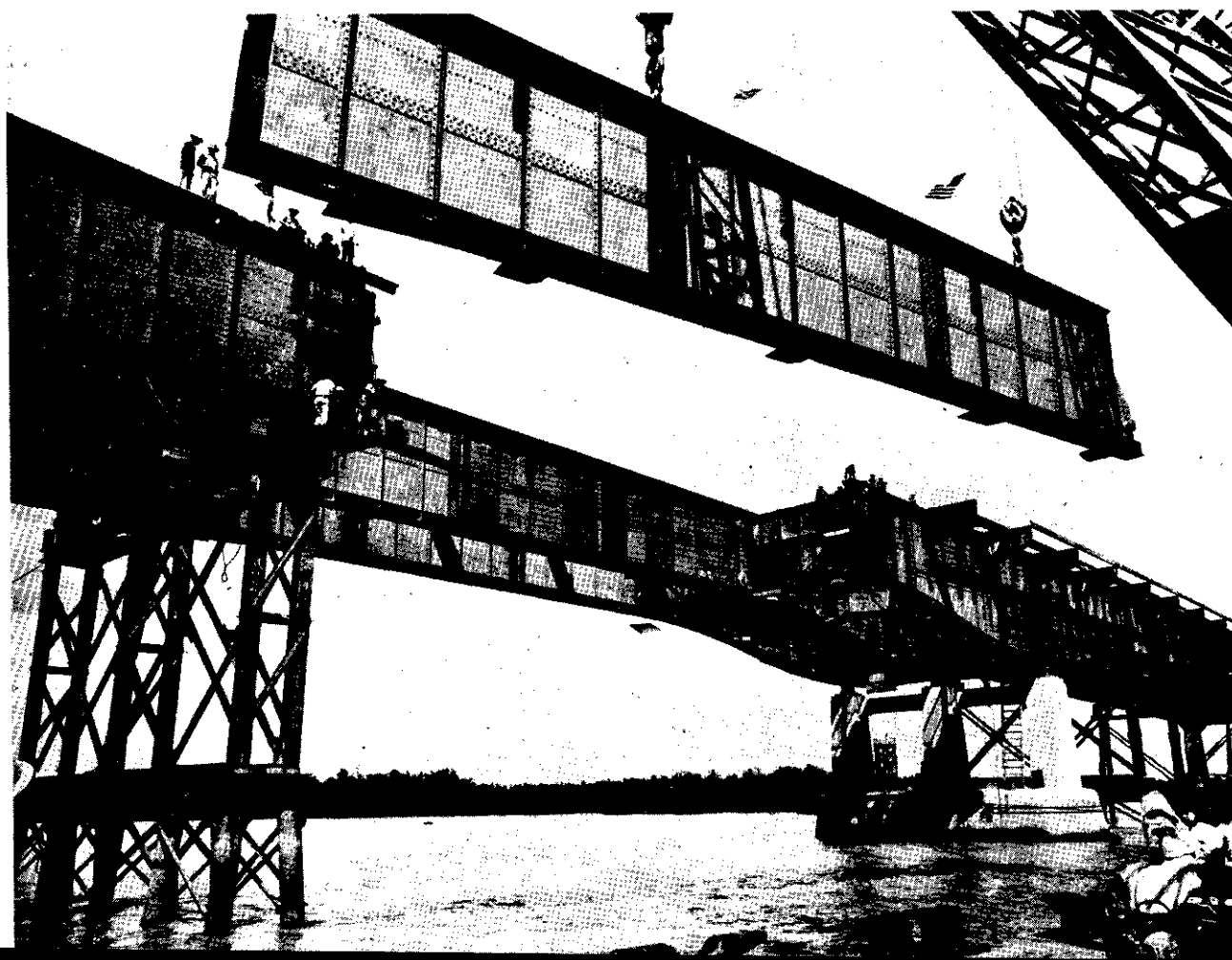
Final steel work on the Saigon River Bridge of the Saigon--Bien-Hoa Highway. This is the longest bridge in Vietnam.
