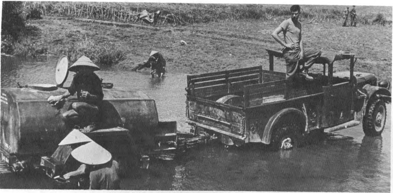
Getting water for construction project
