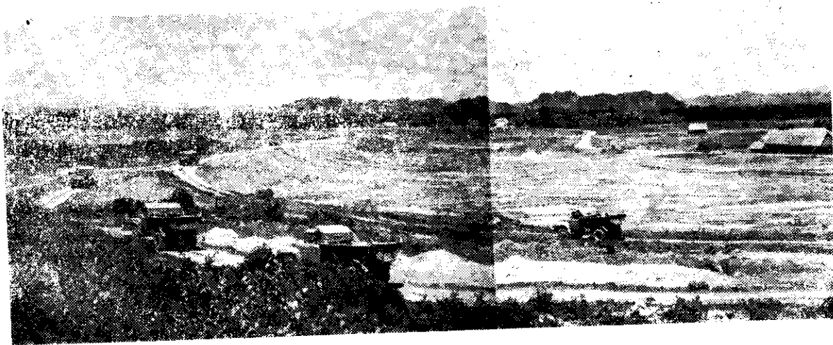
On the construction site of the Yen Quang reservoir (Ninh Binh province)
