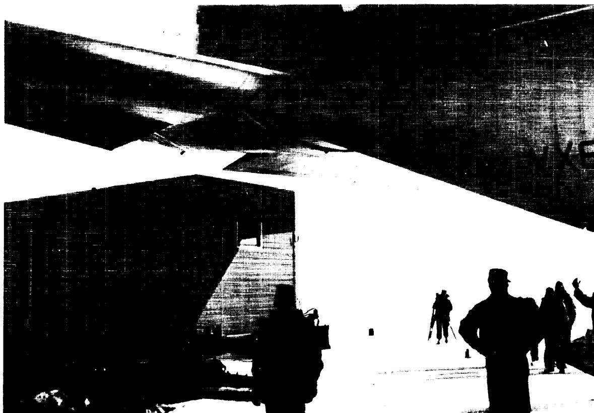
Figure 10. Station module for Eights Station. Eight of these units were interconnected to form the station. Three additional units were established as outbuildings. Modules were fully equipped with collateral equipment and air-transported to the station site 1,384 miles from McMurdo Station.
