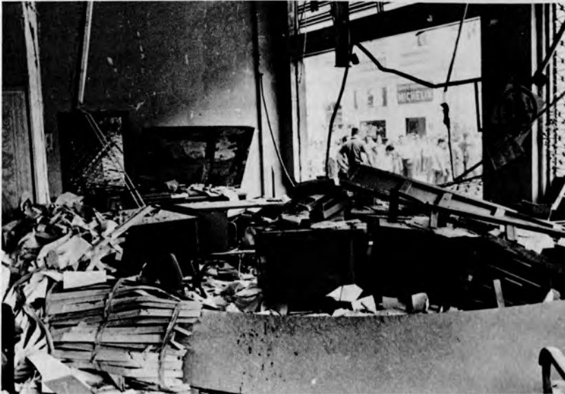
When the U.S. Embassy in Saigon was bombed in 1965, the job of cleaning up the mess, and later designing and building a new, more secure embassy, was primarily an administration and support function.
