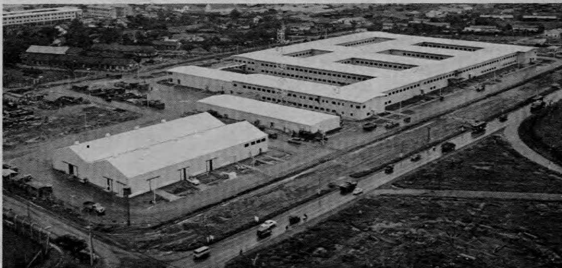
HEADQUARTERS SITE—The new USMACV headquarters building, completed in the latter part of the summer of last year, is located on a 23-acre site at Tan Son Nhut. In a sense, it is a small city as it has its own electric power plant, communications, water wells and sewage system. The two-story building contains the offices of COMUSMACV and his major staff officers. (USN PHOTO)
