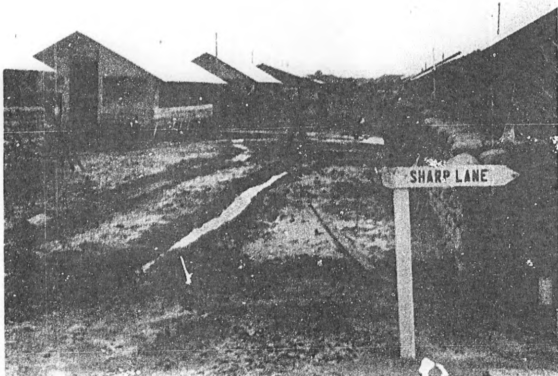
Navy berthing facilities at Dong Tam.
