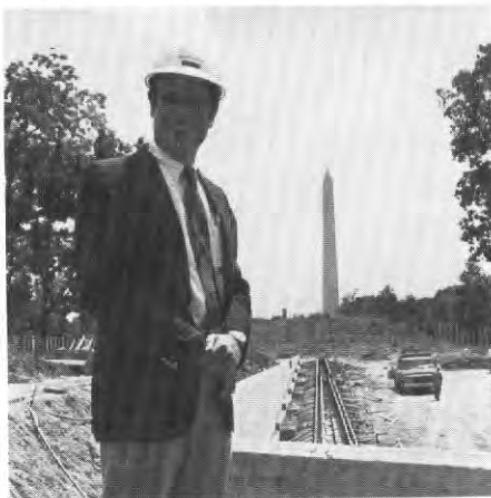
Project Director Robert Doubek making an on-site inspection of construction.
