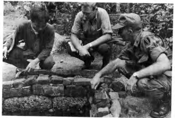
as well as the digging of wells.
