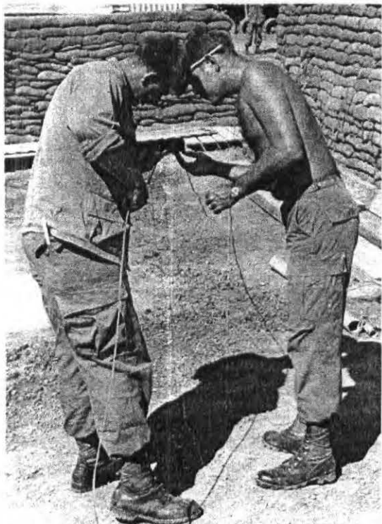
PRECISION —Specialist 5 Jerry Pyles, of Springfield, Ohio (left), and Specialist Ed Szymanski, of East Hartford, Conn., members of the 2nd Battalion, 77th Artillery survey section take a reading from a 30 meter steel tape.
