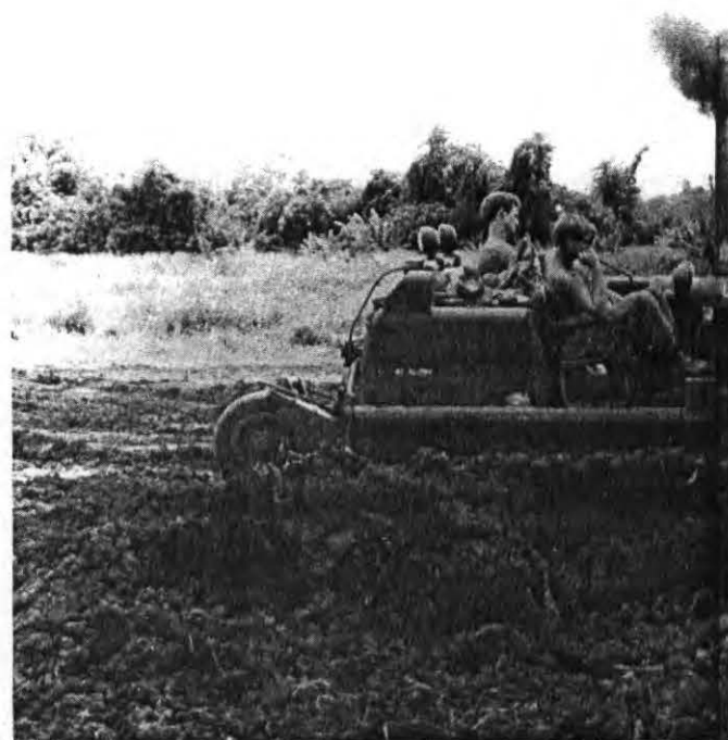
BERM PROTECTION - A bulldozer scrapes up a protective berm at Fire Support Infantry.
