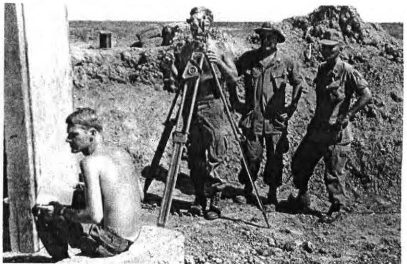
PROPER FIGURES —Specialist 4 Bill Horton, of Greenville, Miss. (lower left), waits for other members of the team to measure the angle between two survey stations, so that he can record the data.
