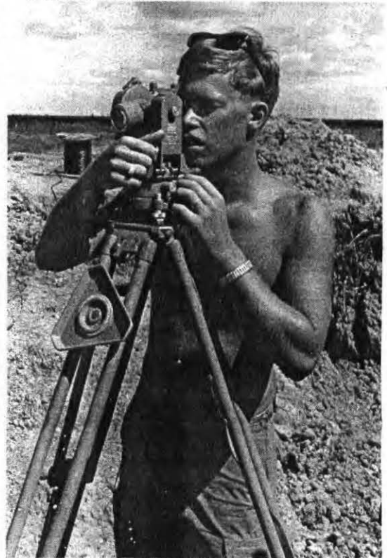
HAIRLINE —Sergeant Bob Forbes, of Iowa City, Iowa, a member of the 2/77 Arty survey section uses a theodolite to measure the angle between two survey stations.
