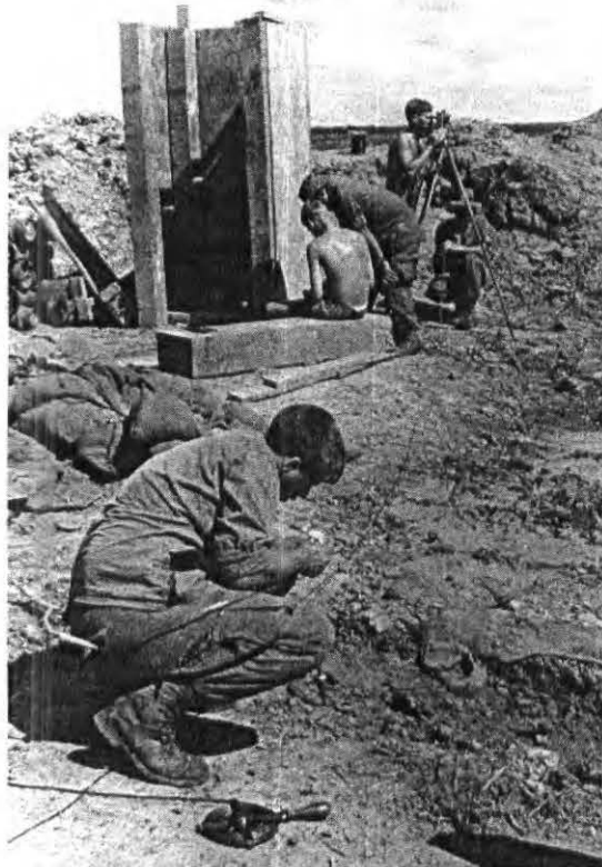
PULLING TAPE —Specialist 5 Jerry Pyles of Springfield, Ohio (foreground), a member of the 2nd Battalion, 77th Artillery survey section measures the distance between two survey stations as other members of the team gather more data.
