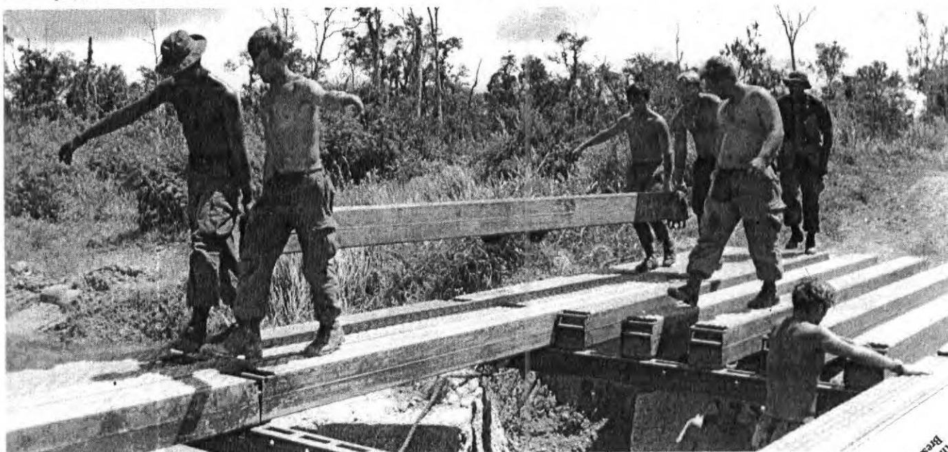
BRIDGING THE GAP — Members of Alfa Company, 65th Engineers construct a 38-foot dry span bridge, eight miles northeast of Nui Ba Den. The frame and the five
