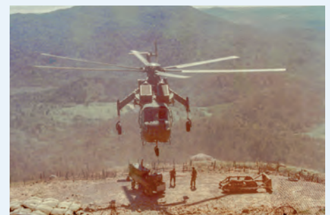
Skycrane helicopter delivering bulldozer
