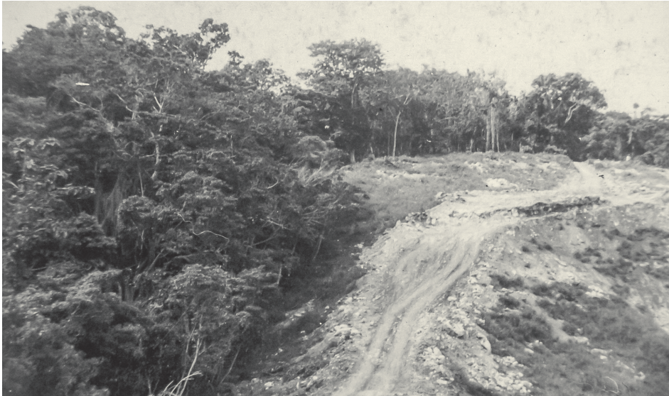
“Wright Road” built by the 57th Combat Engineer Battalion in support of the Mount Austen operations. The engineers pushed the road up and down hills and through the jungles despite the lack of heavy equipment, enduring Japanese sniper fire along the way. The road linked the main perimeter on the coast to the advance positions of the infantry at Mount Austen. The engineers named the road after Lt. Col. William Wright, killed in action in the Mount Austen operation.
