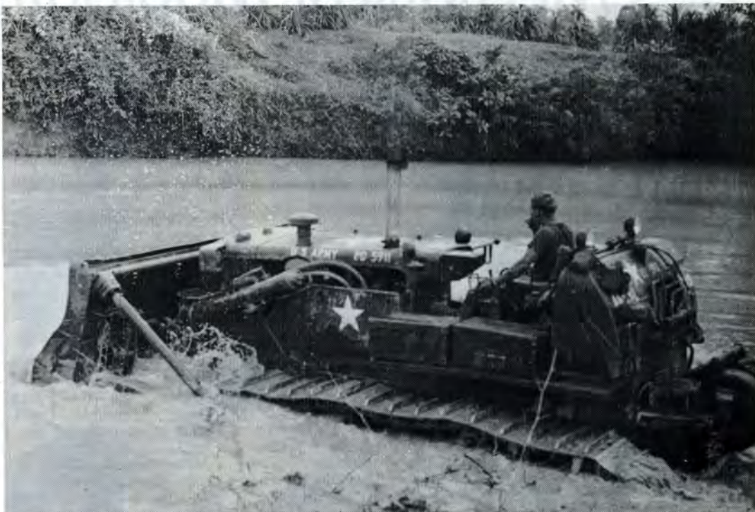
A BULLDOZER PLOWS ITS WAY across a shallow river near Minh Long, about 20 miles northwest of Duc Pho. The 26th Engrs. were constructing a road through rough terrain so self-propelled artillery pieces could reach Minh Long to support division soldiers in the area. (Photo by SGM John R. Spehar, 26th Engr. Bn.)
