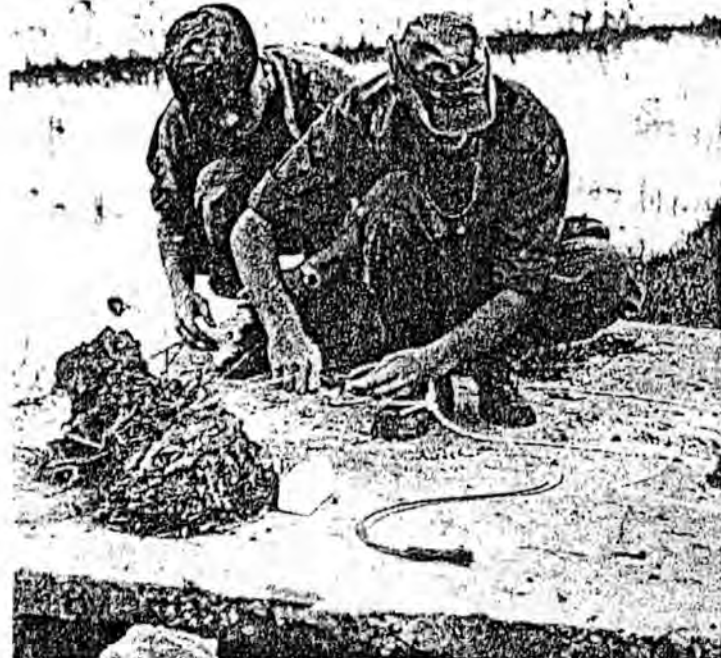
Two demolitions men assigned to the 26th Engineer Bn. carefully place charges of high explosive on the surface of a concrete slab serving as a footbridge on the old Mo Duc Path. When the charges were detonated, the concrete slab and rails were destroyed, but the abutments of the bridge were untouched, as planned.
