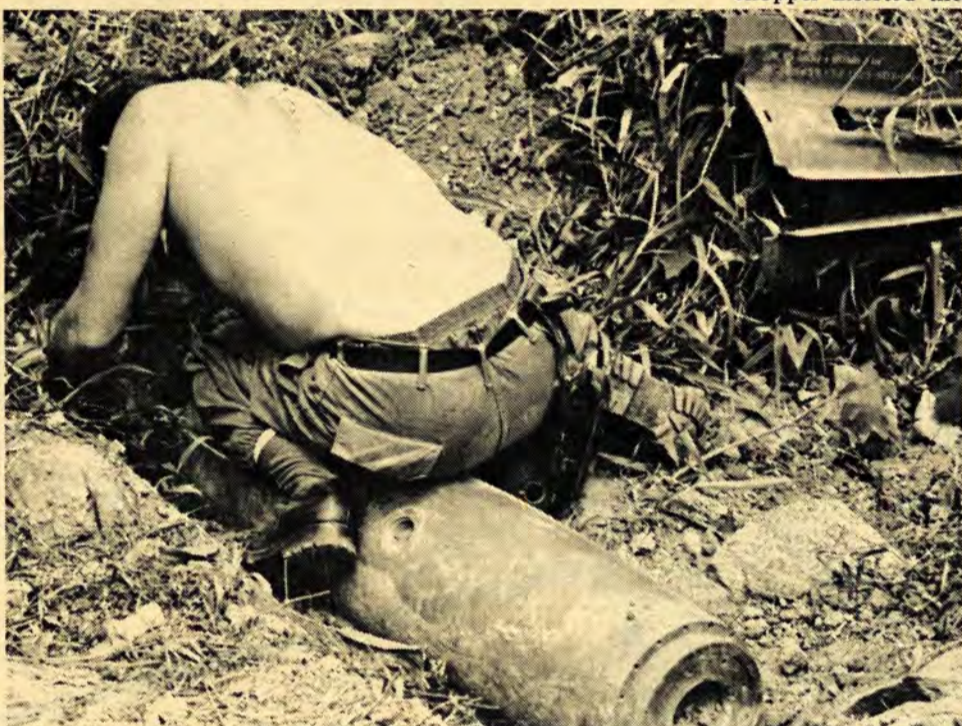
Sergeant Gaddy carefully clears away the dirt from the nose section of the bomb. The discredited tail fin assembly is at left.
