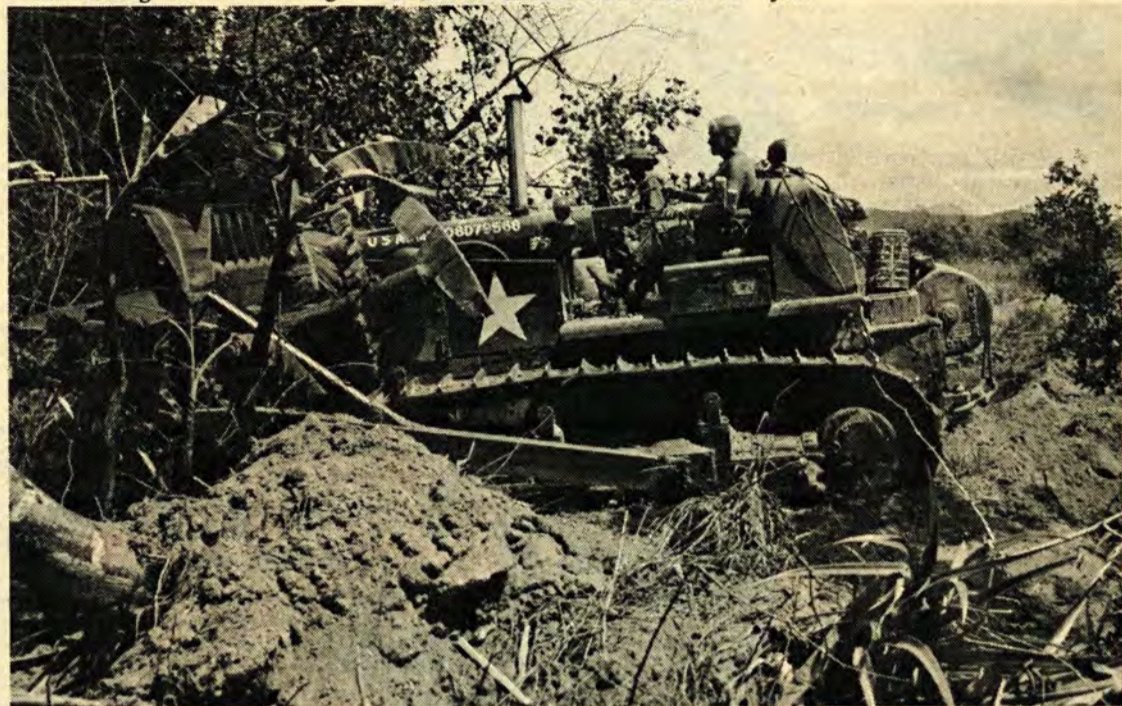
A D-7 bulldozer lumbers forward in search of another chunk of underbrush to munch on. The vehicle is being employed on the land clearing project of the 26th Engineer Battalion five miles northwest of Duc Pho. (Photo by SP4 Peter R. Sorensen)
