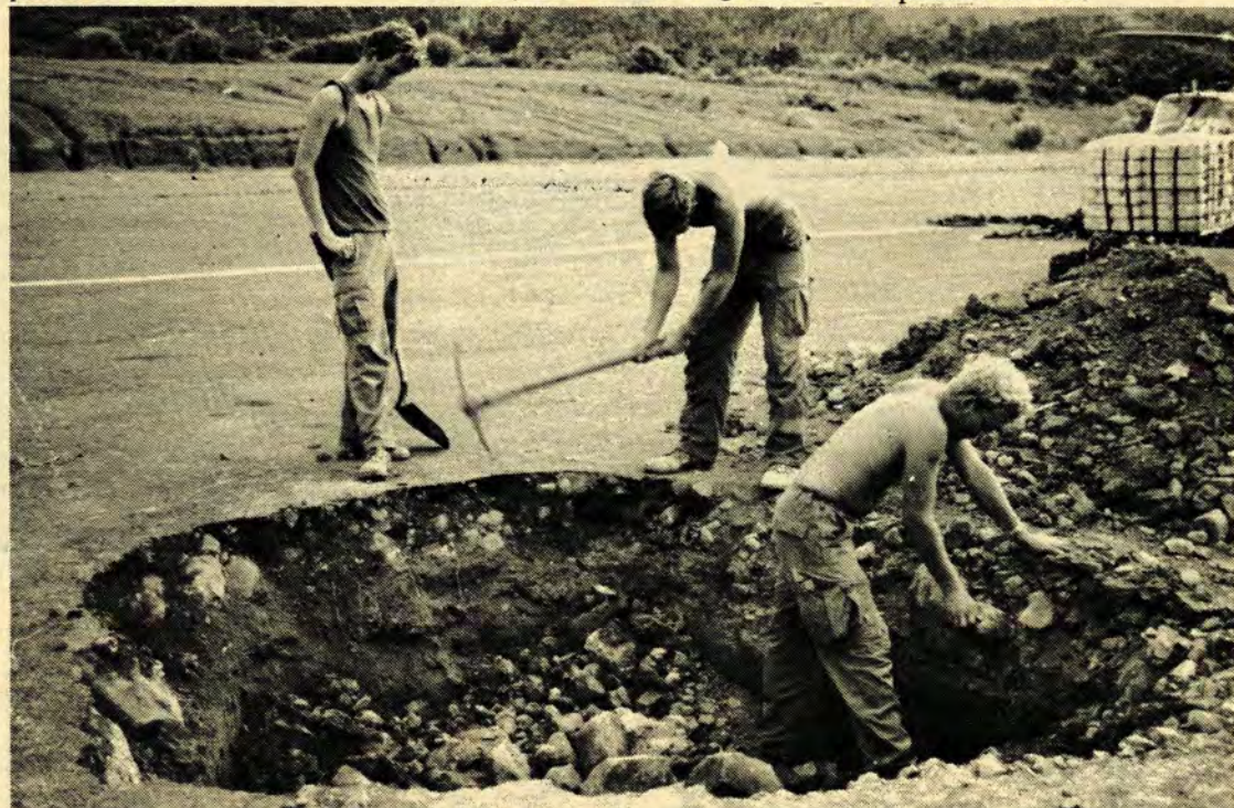
Working under the blazing sun at Kham Duc, these engineers repair the holes in the runway after enemy booby traps were dug out. The Kham Duc runway was recently reoccupied by the Division after its abandonment in 1968. (Photo by PFC Guy Winkler)
