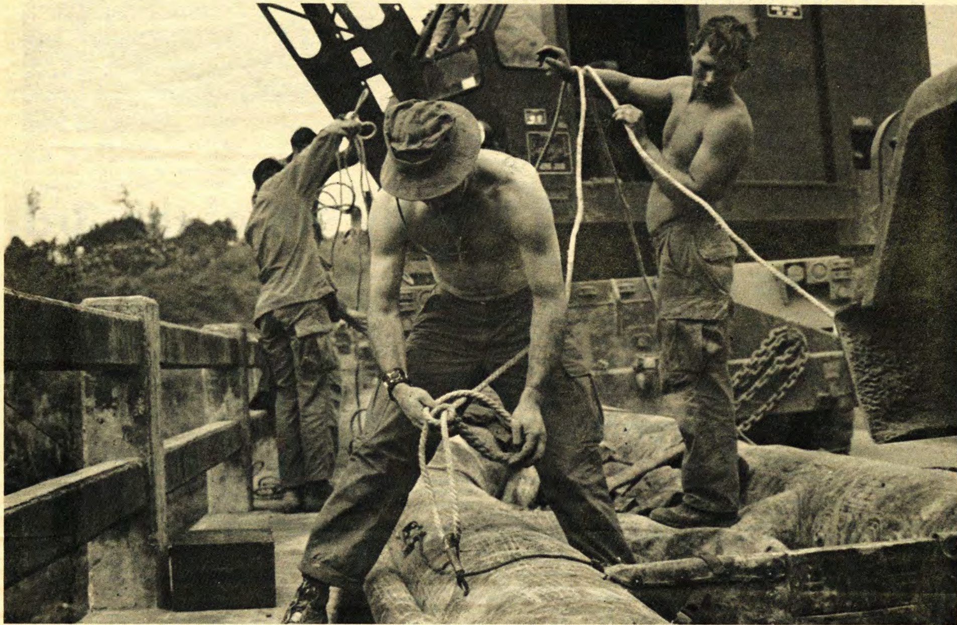
Engineers prepare to hoist a 15 man assault craft over the side of the Quang Ngai Bridge. The craft was employed in assessing mine damage to the supporting piles beneath the 300 foot structure.
