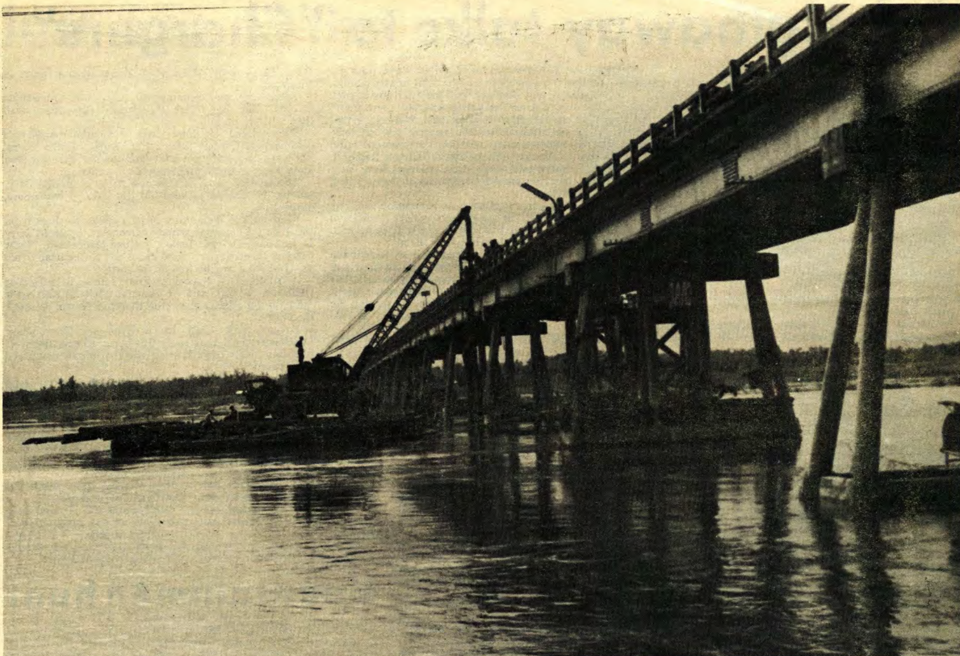
Engineers with the 137th Light Equipment Company drive 60 foot piles into the Song Tra Khuc River, near Quang Ngai. The bridge damaged by a floating mine is being reenforced through the joint effort of Company E, 26th Engineers; Company B, 39th Engineers, and the 137th Light Equipment Company.
