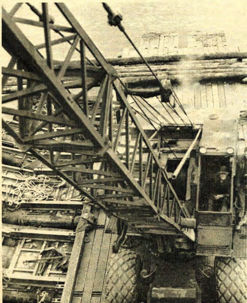
Levers in hand, Specialist 5 Alex Ryan of Charleston, N.Y., guides the crane as it pounds the supporting piles 30 feet below.
