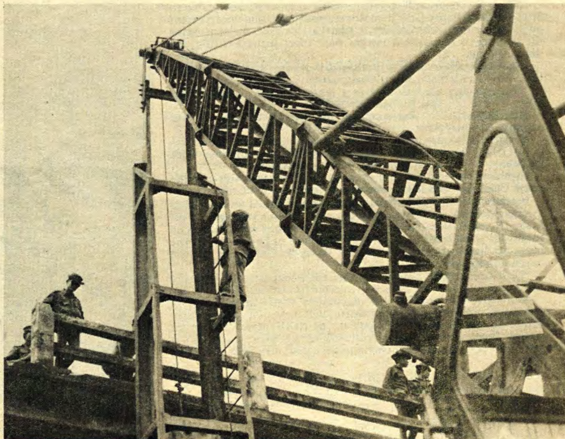
The hefty ruff-terrain crane lowers the boom on the 60 foot piles in the construction project.
