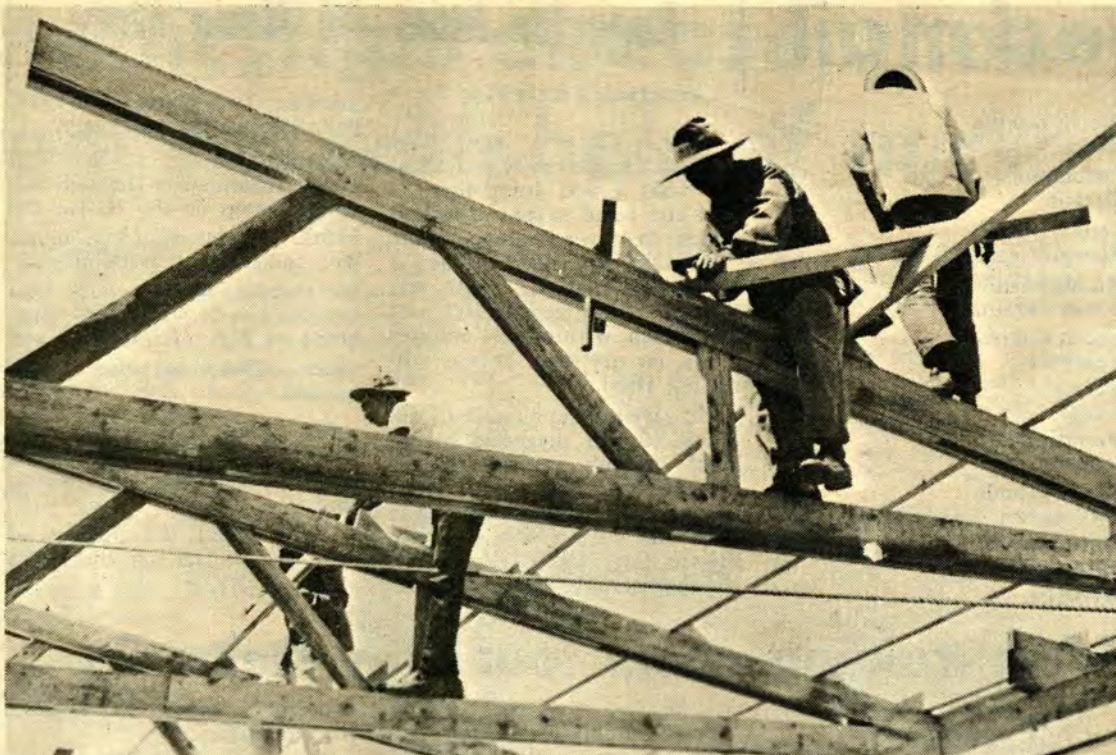
Four Korean workmen put finishing touches on the roof supports for the Officers Club roof. The roof, finished with tin, replaced the thatched roof which blew off during a May typhoon. (U.S. Army Photo by Sp/4 Ron Cryderman)
