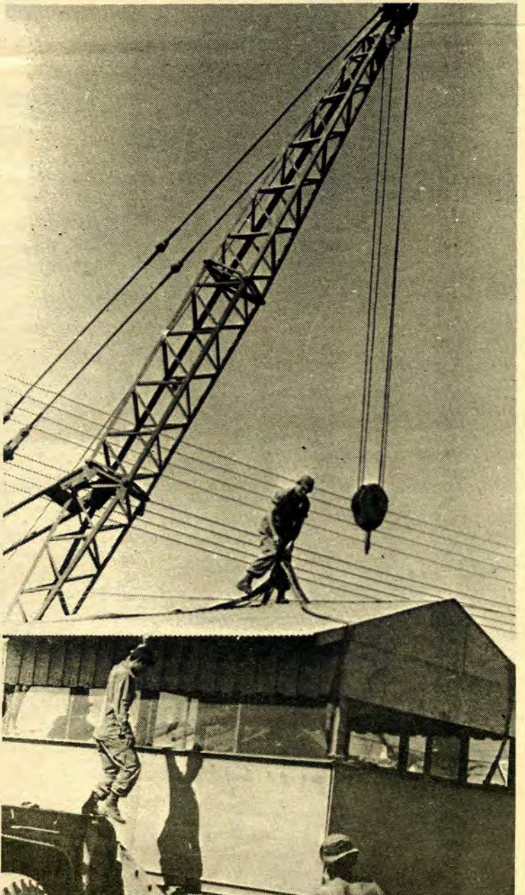
A new office building gets emplaced at 23d Infantry Div (Americal) as engineers prepare the hoist to lift the hootch from a flatbed trailer. (U.S. ARMY PHOTO BY SP4 SAM ROUSSO)
