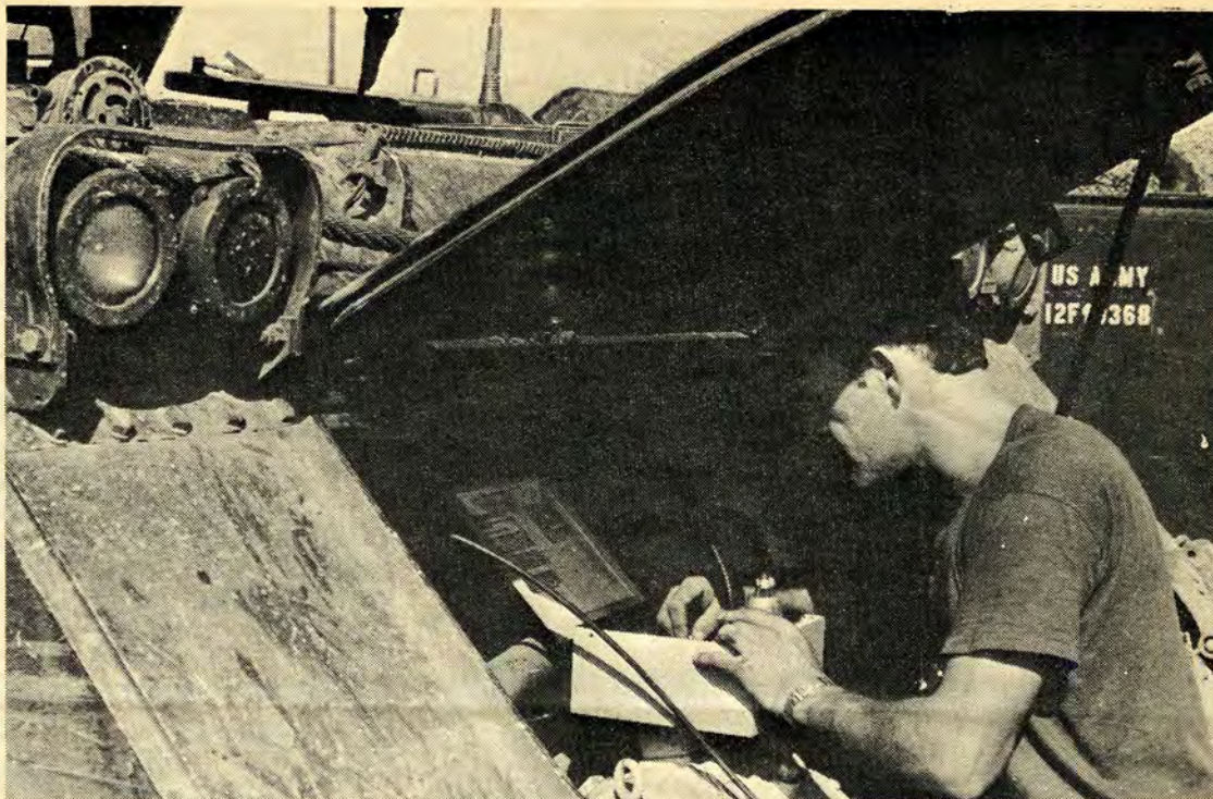
CHECKING IT OUT—Staff Sergeant Joseph A. Decilles checks out the charging system in this M113A1 Armored Personnel Carrier. Decilles
