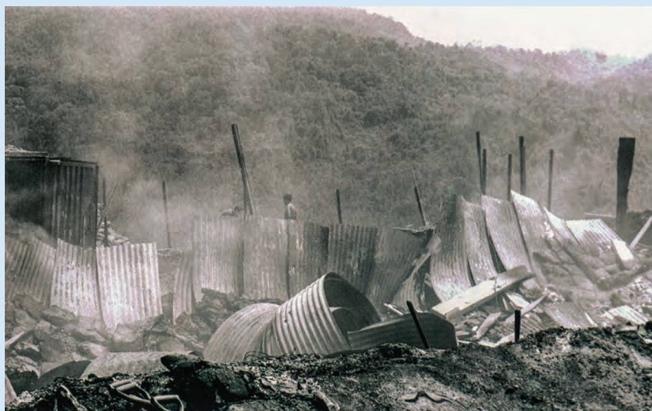
Wooden battalion TOC bunker burned to the ground. Metal sheeting on roof collapsed into the excavation. Culvert halves formed a guard position on top of the TOC.
