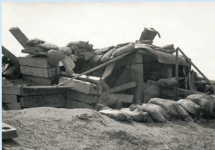
Damaged bunker. Bunkers were pre-fabricated of heavy wooden beams in Chu Lai and flown by heavy lift helicopters to Mary Ann. Earth filled ammo boxes and sandbags were used for protection.
