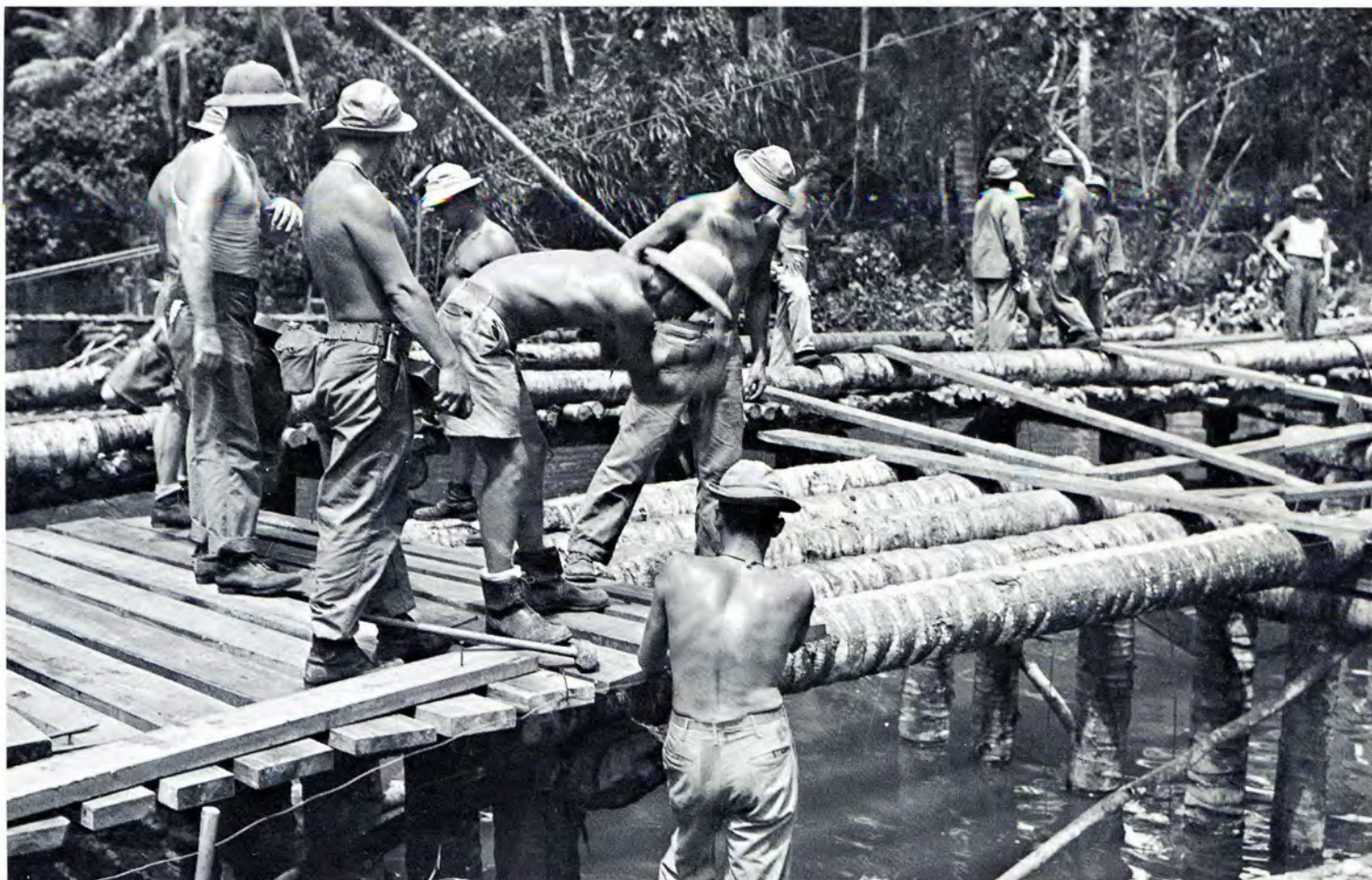
Engineers construct bridge on Guadalcanal.
