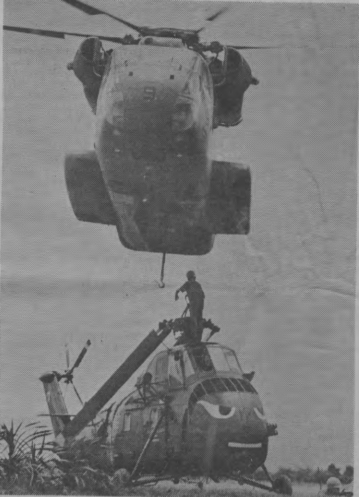
TEAM EFFORT —A CH-53 Sea Stallion from Marine Heavy Helicopter Squadron-463 prepares to lift a downed UH-34 from a landing zone. The lift was successful despite enemy fire directed at the CH-53 and Cpl. Claude H. Anderson, 19, (Atlanta, Ga.) of the recovery team, waiting to make the hook up. (Photo by: Sgt. Rich Groscost)
