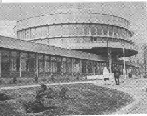
The new cultural centre at Vac.
