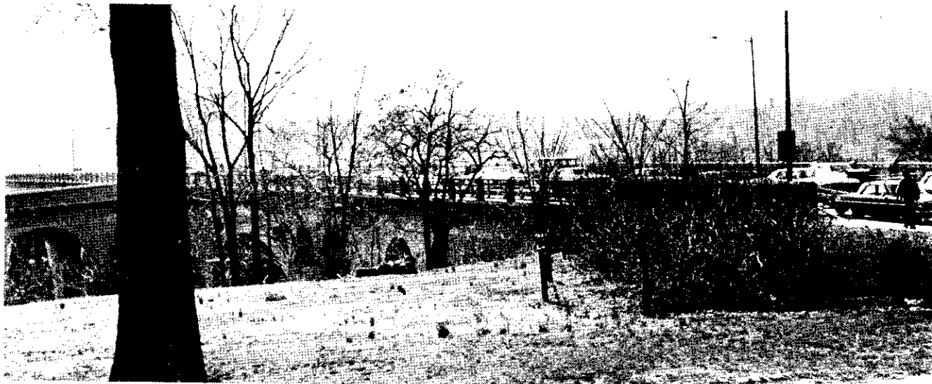
Key Bridge, filmed from the D.C. Side of the Potomac. The open area lies adjacent to "M" Street, leading to Georgetown. Not visible, but traveling beneath Key Bridge is Whitehurst Highway.
