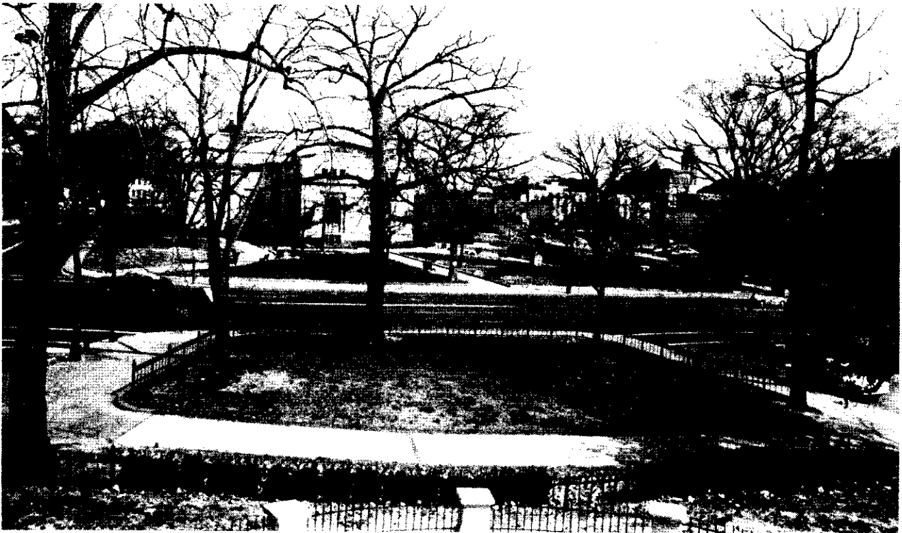
Mt. Vernon: facing east, the D.C. Public Library can be seen between Massachusetts Avenue, on the left and "K" Street on the right.
