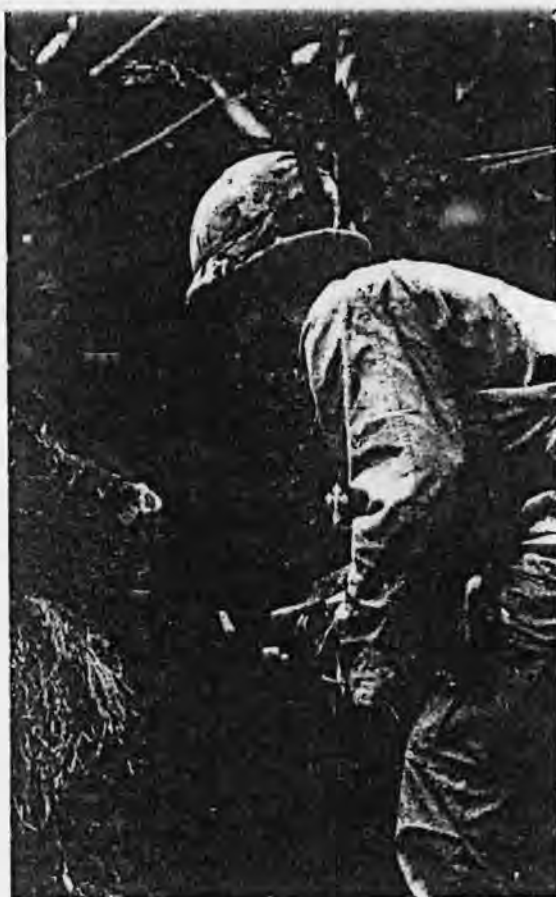
'Charger' cautiously enters tunnel
