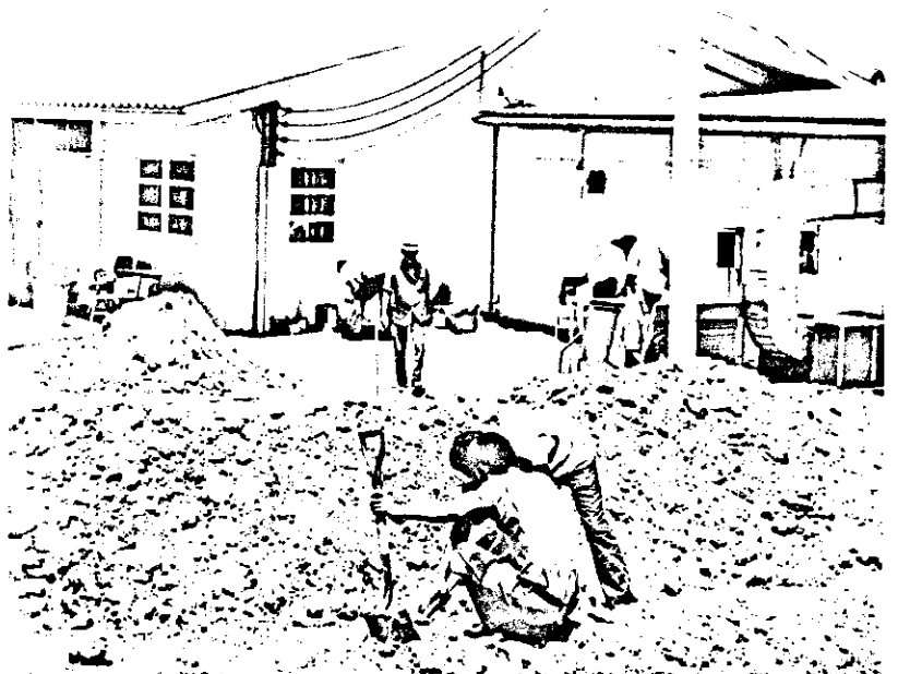
CONSTRUCTION HAS FINALLY BEGUN for the expansion of the NCOOM's Ballroom.
