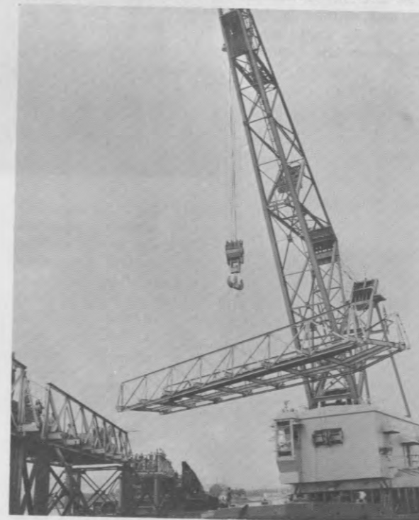
NSA crane lowers new span into position.
