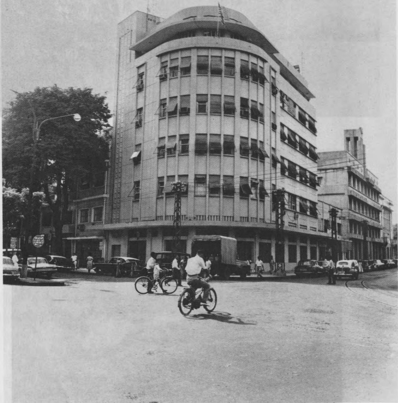
EMBASSY - MAIN BUILDING
