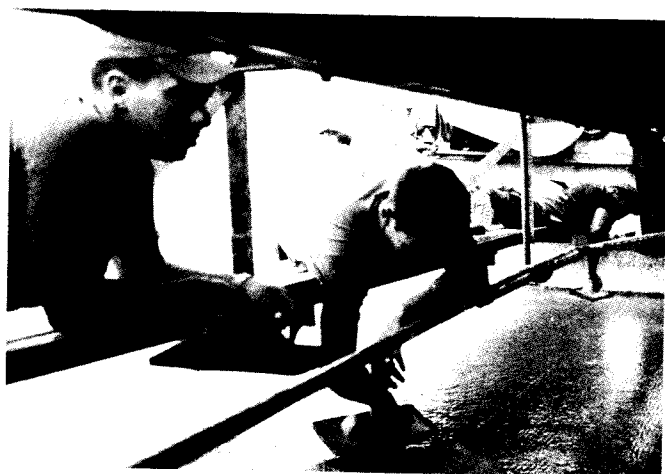
(Above) Men of the 937th Engineer Group, using floats and draped over the "running board" of a paving machine, put a smooth finish on a concrete slab near An Khe. (US Army Photo)
