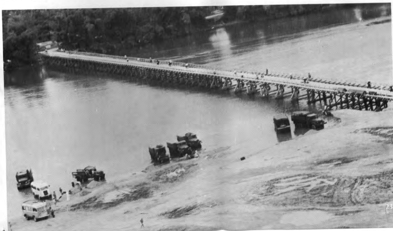
The Dien Khanh bridge, its superstructure completely washed away by the flooding Song Cai River as it stood November 30, 1967, and the completed span, less than 100 hours after the 864th Engineers began construction. The bridge now insures a safe crossing point for military and civilian traffic using the Nha Trang Bypass, a vital link in HL 1 between Cam Ranh Bay and points north.
