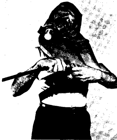
Figure 9331-6. Inflatable life preserver for use by submarine personnel.
