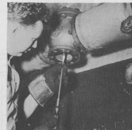
Grinding Main Valve
