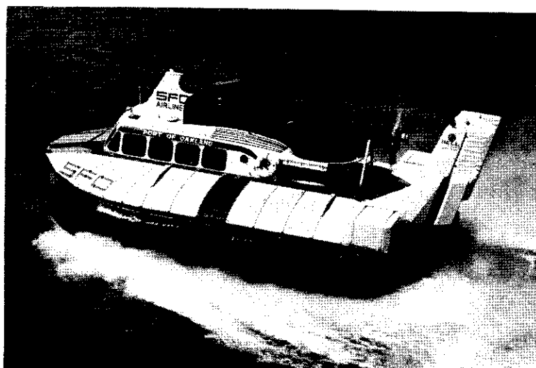
The Hovercraft is certificated for speeds up to 50 MPH. Note turbulent water surface, but very little wake.
